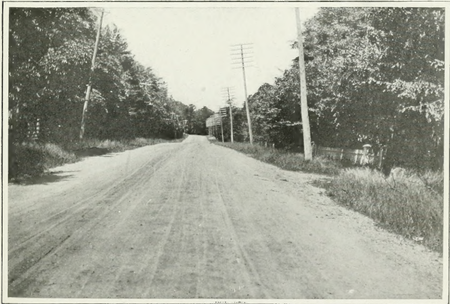
Dundas Street, near Toronto. Carpeted with tar and fine gravel.
